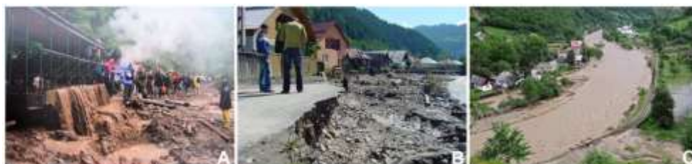
Fig. 4. The effects of the flood, 2008: A) „Mocănița” blocked on vaser Valley; B) Affected infrastructure; C) Flooded floodplain (source: A - Michael Schneeberger, 2011; B, C - www.emaramures.ro , 2008).
