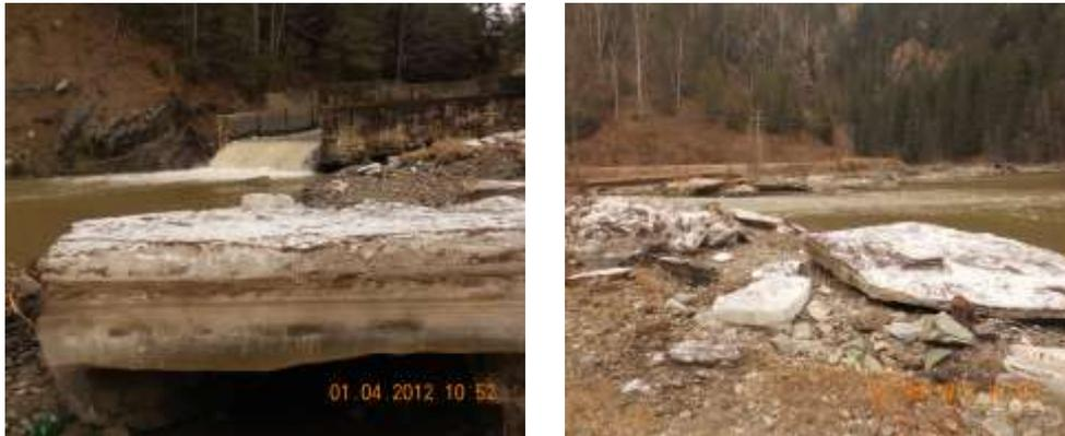
Fig. 4. Massive ice fragments brought from Ortoaia (upstream Zugreni dam) that have passed over the shuttle, remaining on land at its base (ice thickness and stratification can be observed), 01.04.2012
