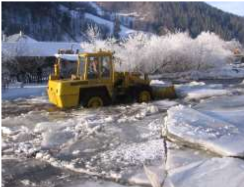
Fig.6 B. Works of removing ice jams from the Bistrița floodplain, (photo Gavril Petrică)
