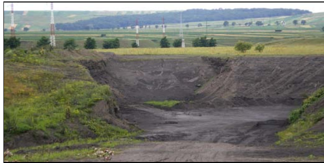
Fig. 2. Highly uneven terrain at TERMICA ash landfill. (April 2010)
