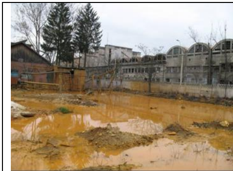
Fig.12 – Săsar mine – mine water evacuation plant
