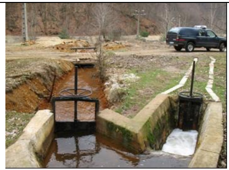
Fig.13 – Nistru mine – water treatment plant at Câmpurele
