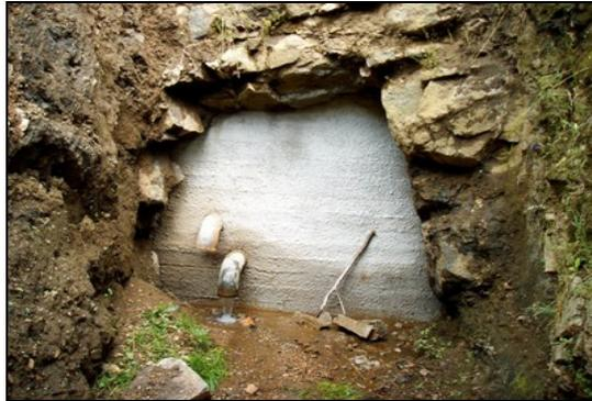
Fig. 3 - Gallery 10, Pietraru enclosed by concrete walls provided with drainage pipe (Source: [www.geolex.nextra.ro](http://www.geolex.nextra.ro))
