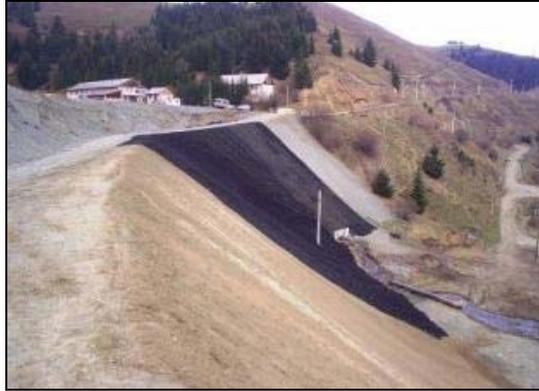
Fig. 2 - The dump of Jolotca mining during the works of greening with poly cells
