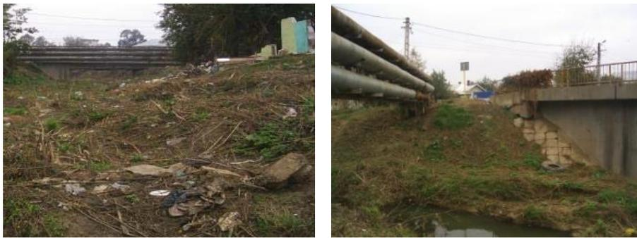
Fig. 13 – The heavy concrete bridge and nearby central heating ducts that effectively blocked the flow of the flash flood
