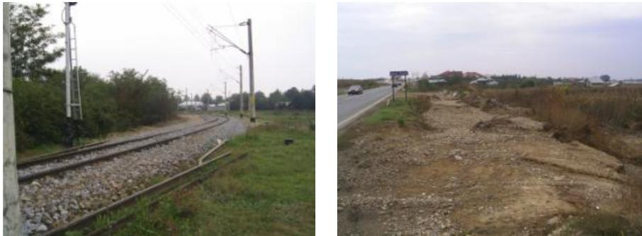
Fig. 11 – Erosion of the embankment of the Barlad-Tecuci railway (which needed urgent repairs for a distance of 300m) and that of the DN24, both man-made structures forming a temporary dam in the flood path
