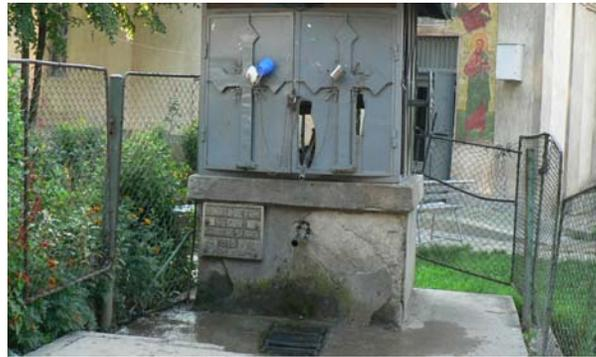
Fig. 4 - The metallic reinforcement that protects the fountain with elevator cups situated in Bukovina Street of Botosani
