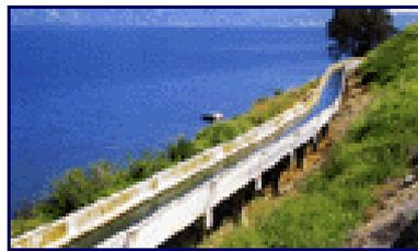
Fig. 5 - Open sector of the National Carrier (line II) that captures the salty springs on the western shore to the Dead Sea
