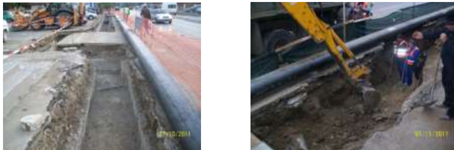
Fig.4. Works which affects the vegetation performed on Mihai Eminescu Boulevard
